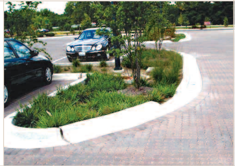
Figure 25: Planting islands with depressed curbs allow stormwater to run from paved areas into the islands.
