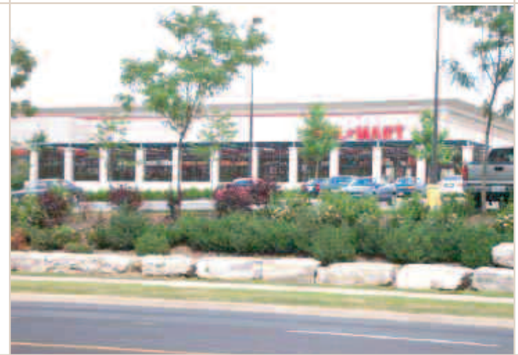
Figure 19: Landscaped low walls help screen the parked cars while allowing visibility to the area.
