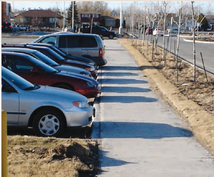
Figure 11: This walkway permits unobstructed pedestrian movement from the store entrance to the public street.
