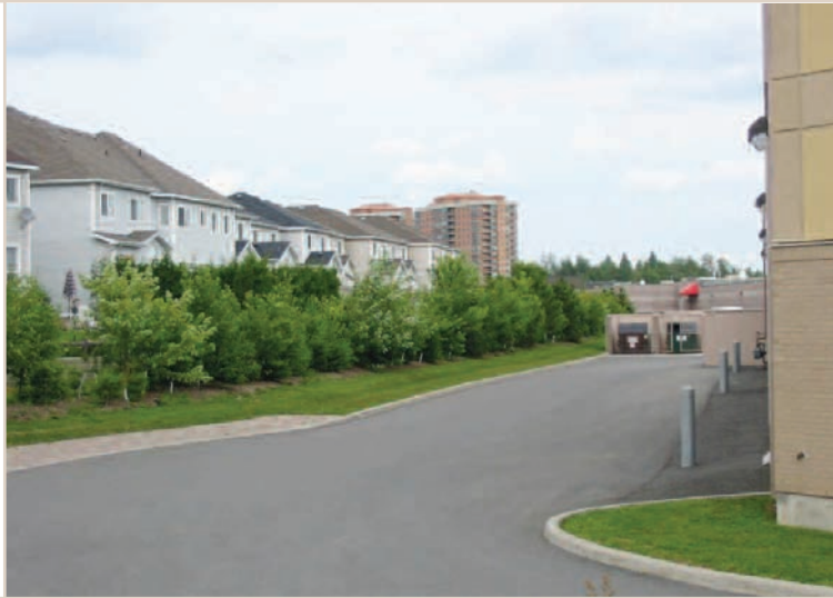
Figure 22: Landscaped buffers provide an appropriate transition between large format retail sites and residential areas.
