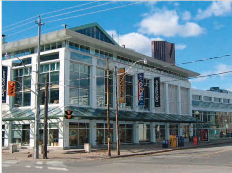
Figure 14: Glass awnings on this building protect pedestrians from the weather.
