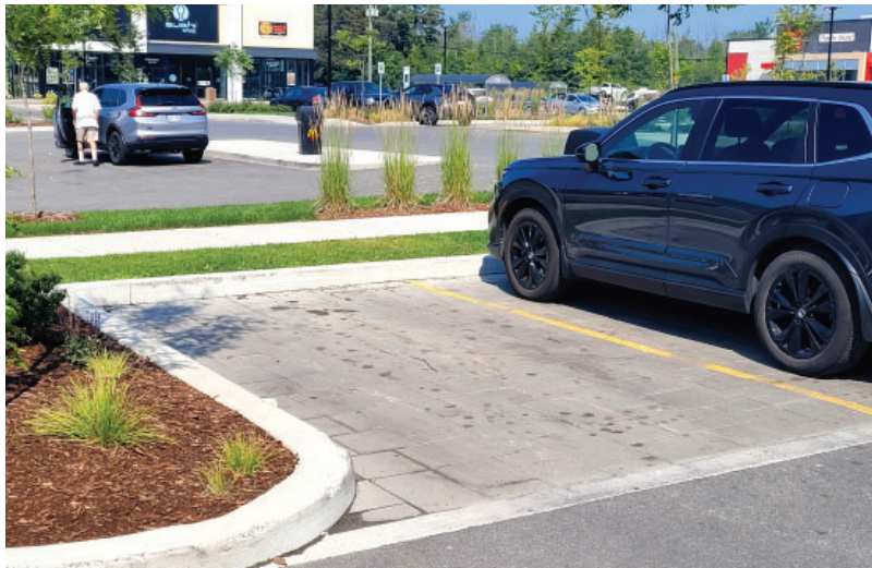
Figure 35: Use of permeable pavement in the parking area increase water penetration.
