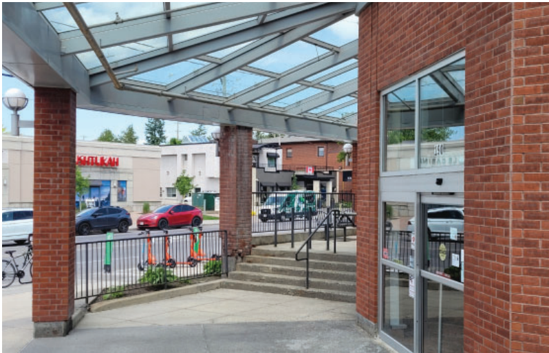
Figure 5: Glass awnings on this building protect pedestrians from the weather.
