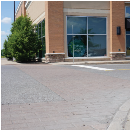
Figure 7: Minimal grade changes and conflict points with vehicles create a comfortable pedestrian environment.
