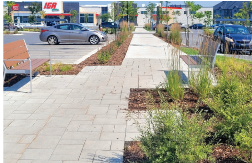
Figure 36: Use of permeable pavement and soft landscaping in the pedestrian walkway adds visual interest and also mitigates stormwater runoff.
