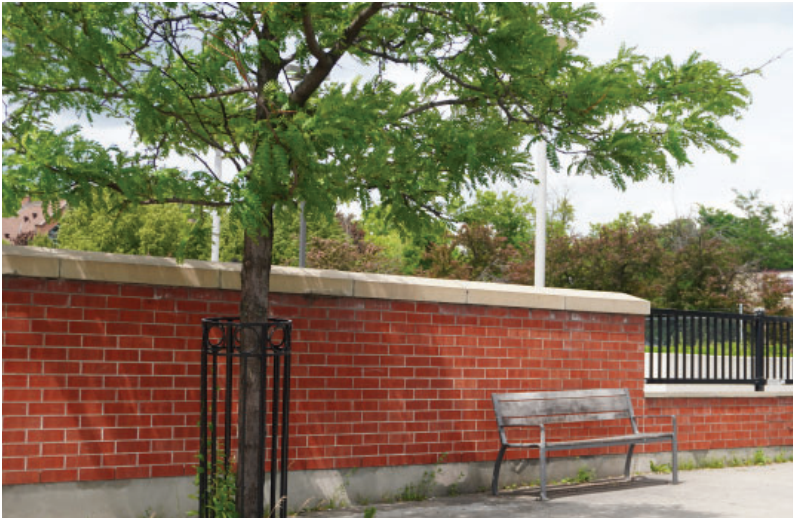
Figure 25: The solid brick wall establishes street edge and screens parking from the street.
