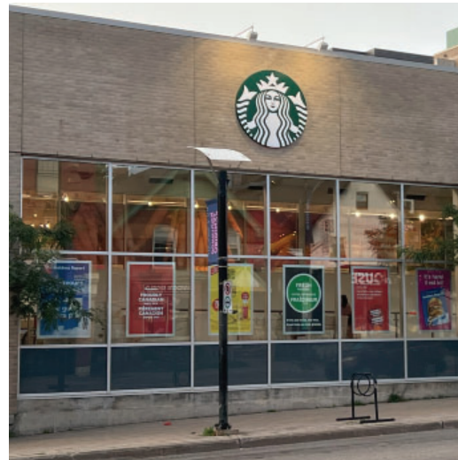
Figure 3: The main façade of this commercial building faces a public street and has over 60% transparency.
