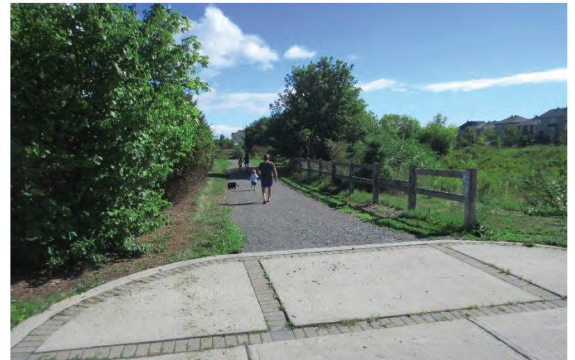
Figure 33: This pathway intersects the sidewalk.
