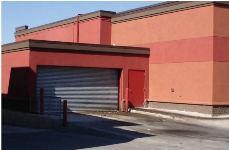
Figure 70: This building features an enclosed structure for garbage, loading and service areas that are accessed from the rear of the building. The enclosed service areas allows for a more visually appealing front along the streetscape
