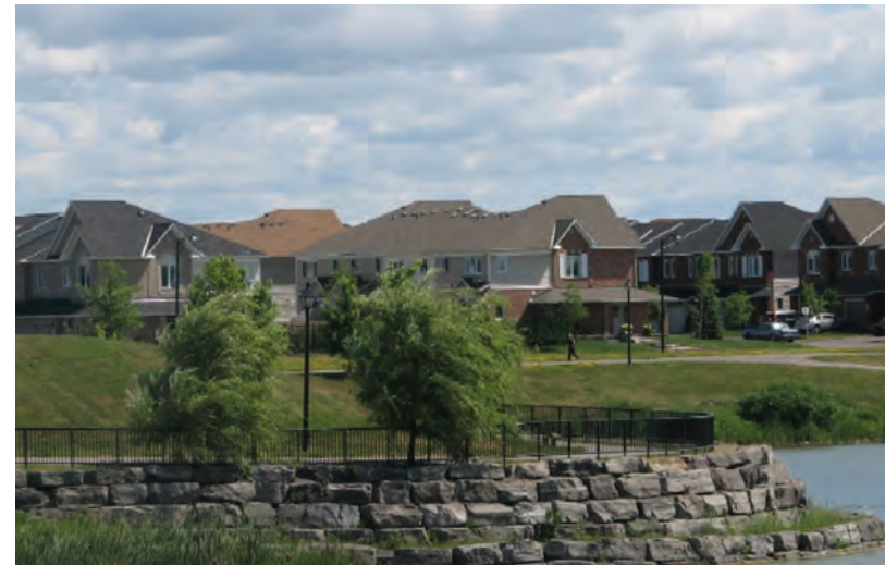
Figure 38: The fencing around this stormwater management pond fits with the overall design of the amenity and contributes to safety.
