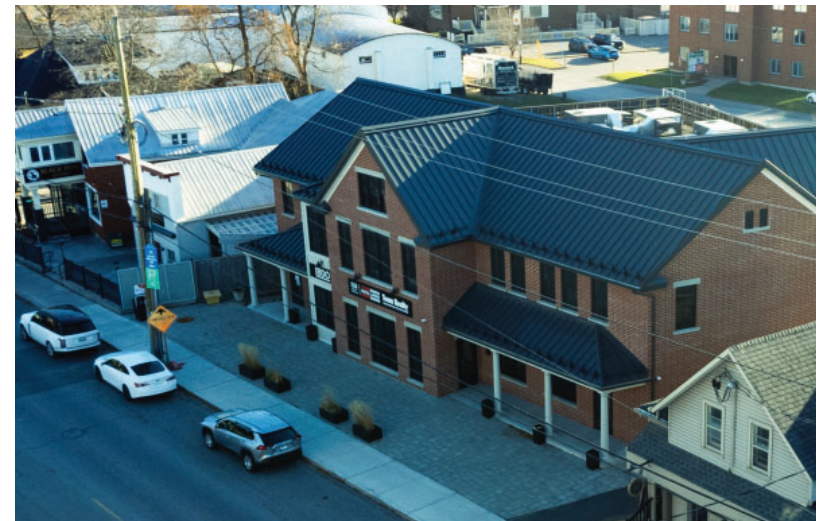
Figure 11: New development provides proper transition and maintains the built form character of the village. (Manotick)
