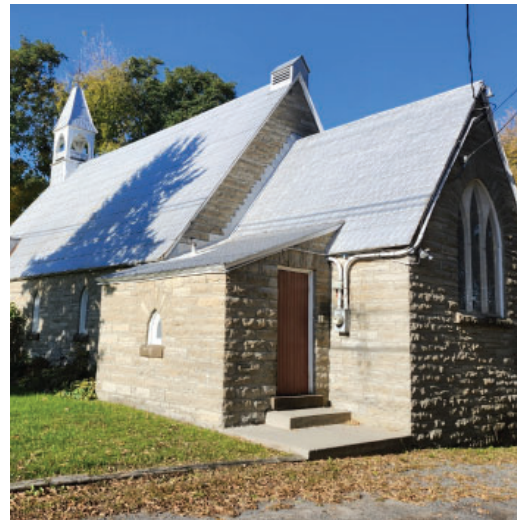
Figure 13: A former church currently operates as Ottawa Public Library branch. (Munster)
