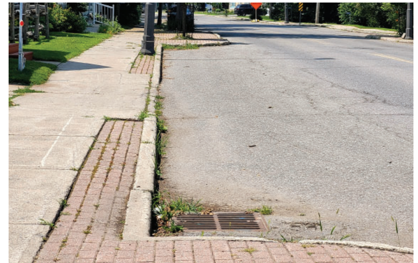
Figure 24: Sidewalks in a village core contrast the roadway and help define the pedestrian area. (Cumberland)
