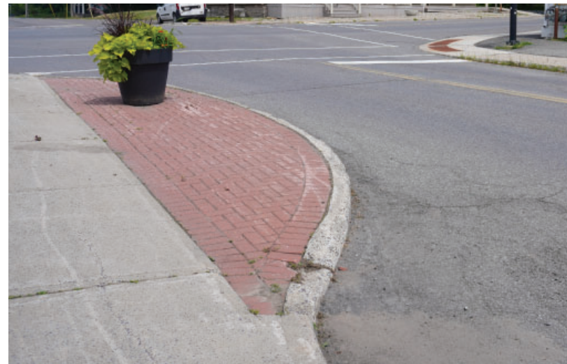
Figure 32: Curb extensions and change of materials at the street intersection in village cores and along main streets support traffic calming.
