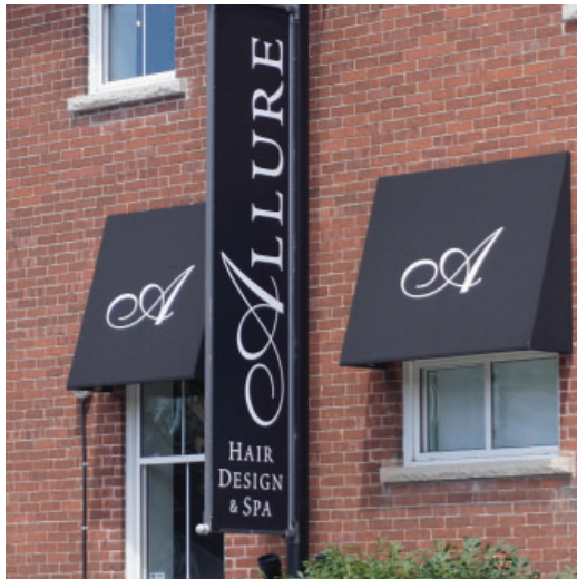
Figure 25: Use of awnings in the commercial building facing the street. This adds element to the pedestrian realm.
