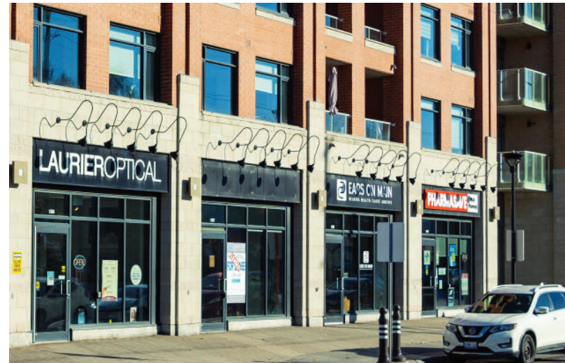
Figure 19: Task oriented sign illumination avoids glare.
