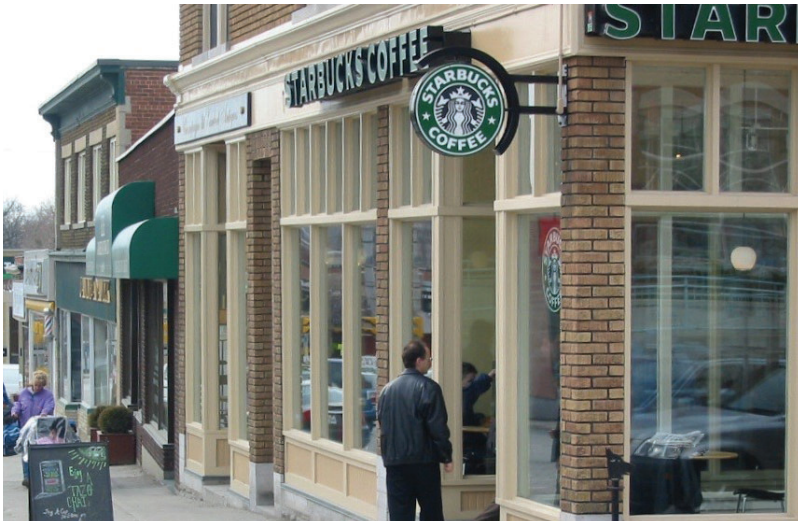
Figure 18: Compact signs fit in with the design of the building.
