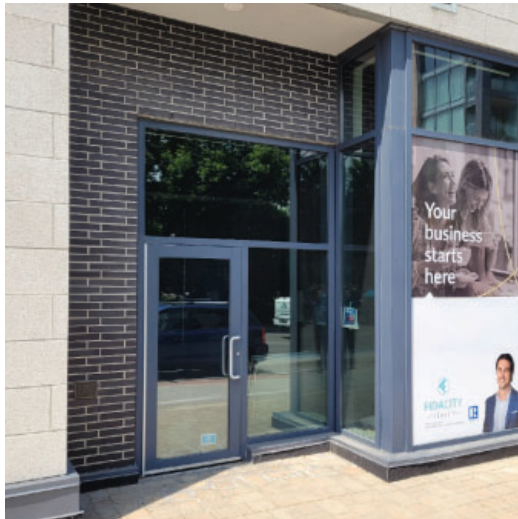
Figure 3: Accessible entrances of the commercial units that are recessed to ensure the sidewalk is unobstructed.
