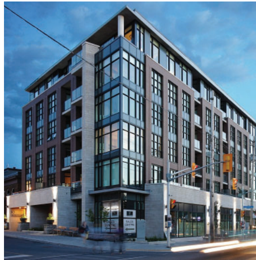
Figure 16: Architectural detail enhances the streetscape on the public sides of a corner building.
