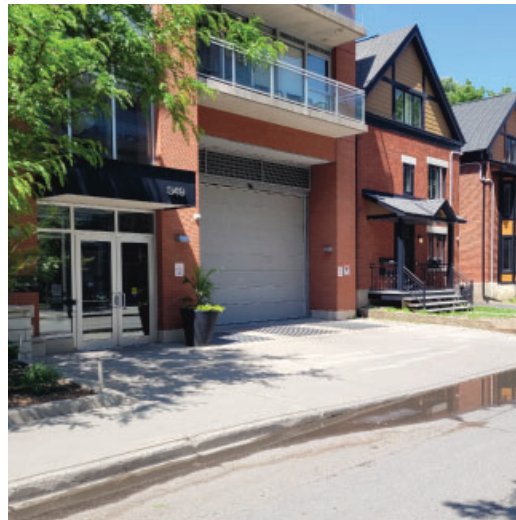
Figure 8: This development internalizes loading and garbage collection facilities.
