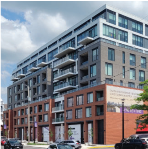
Figure 10: Buildings set back above 3-4 storeys preserve a human scale and allow more light to reach the sidewalk.
