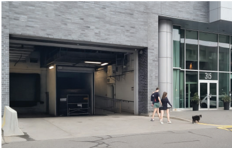
Figure 17: The waste collection area enclosed within the building is screened from the public view.
