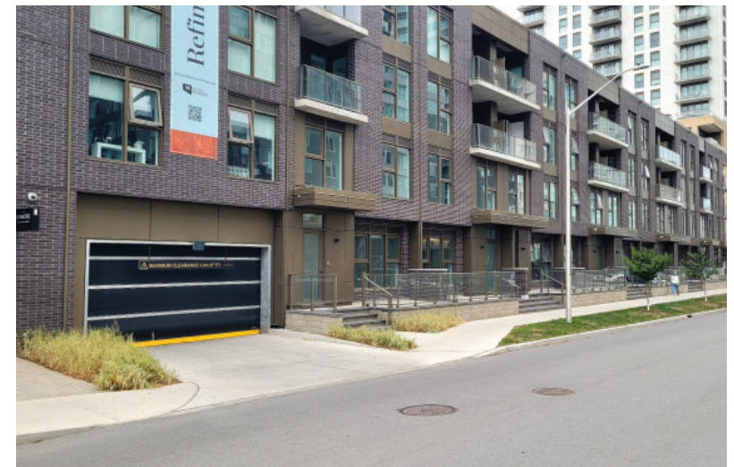
Figure 16: On large sites, loading zones can be located underground to minimize impacts on pedestrians and cyclists. Pedestrians and cyclists should be clearly visible from the loading ramp exit.
