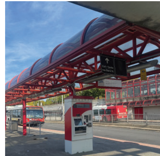
Figure 44: The Billings Bridge Plaza is connected to the Transitway via several covered pedestrian walkways..
