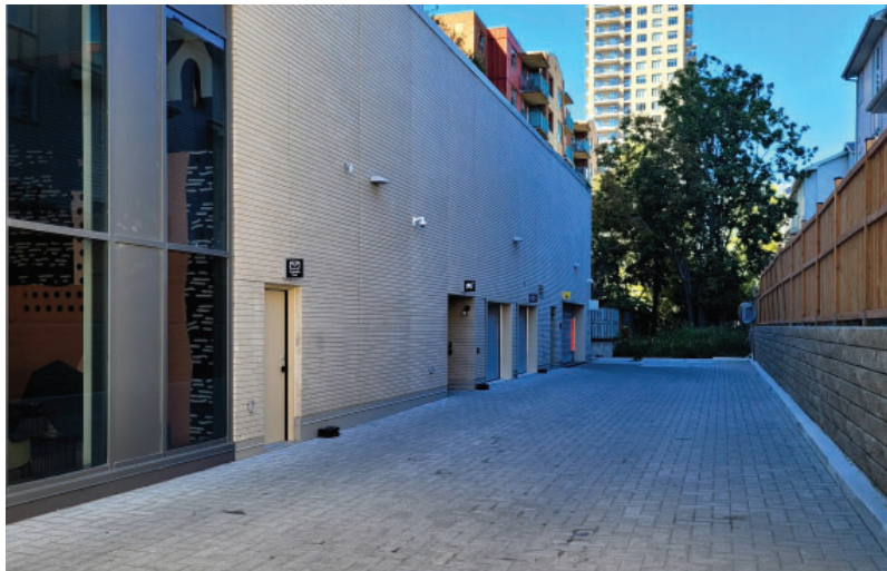
Figure 15: This loading area is located off the street and within the building, which helps to minimize disruptions to pedestrians, cyclists, and other vehicles.
