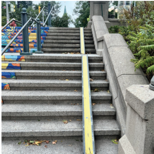
Figure 9: Bicycles ramps on staircases help to facilitate enhanced mobility for cyclists.
