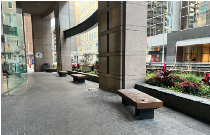
Figure 38: The colonnaded pedestrian space has sufficient height and width to accommodate pedestrian volume.
