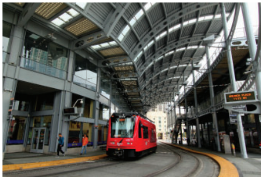
Figure 1: American Plaza in San Diego is an example of a mixed-use TOD building with uses geared towards both local and non-local residents alike, featuring office space (49 000 m 2 ), retail (2000 m 2 ) and a museum (1000 m 2 ).
