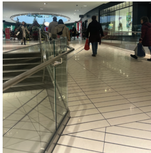
Figure 36: A ramped floor with gradual level changes that meet accessibility requirements is preferred over stairs.
