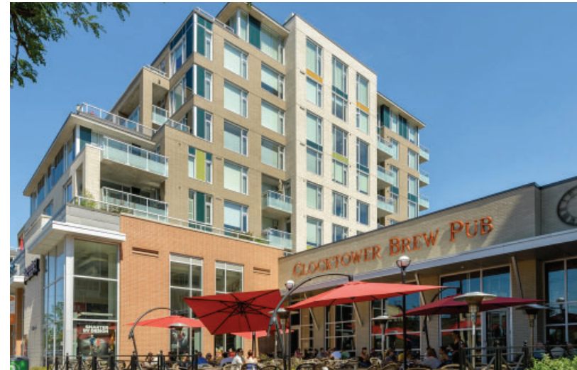
Figure 19: Building with setbacks above 4-5 storeys minimize massing and shadowing impacts on the public realm and allows more light to reach sidewalk.
