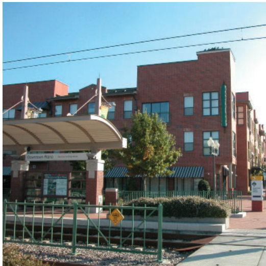
Figure 5: The Plano transit station in Dallas, Texas includes a mixed-use complex between the station and the parking garage to provide passengers who utilize this Park & Ride with a short, attractive walk featuring amenities such as street-level retail.
