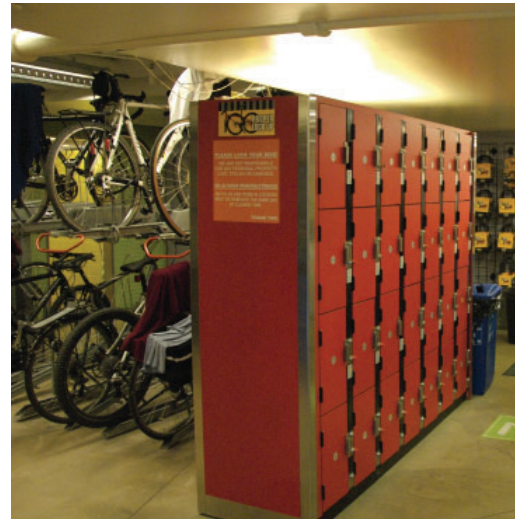
Figure 10: Transport Canada recommends one shower per 100 employees as a good ratio for providing showers and change room facilities in the workplace.
