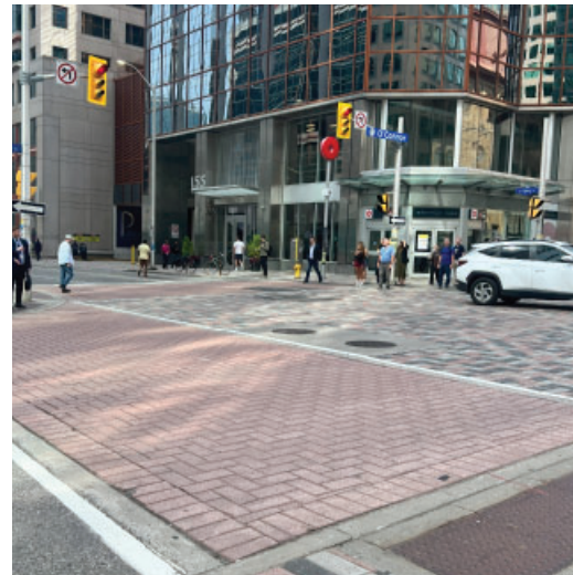
Figure 40: This pedestrian crosswalk at Parliament O-Train Station is made from pavers, which makes it stand out from the roadway asphalt.
