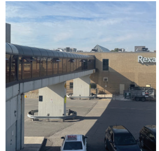
Figure 41: Billings Bridge station provides a grade separated pedestrian connection to retail services.
