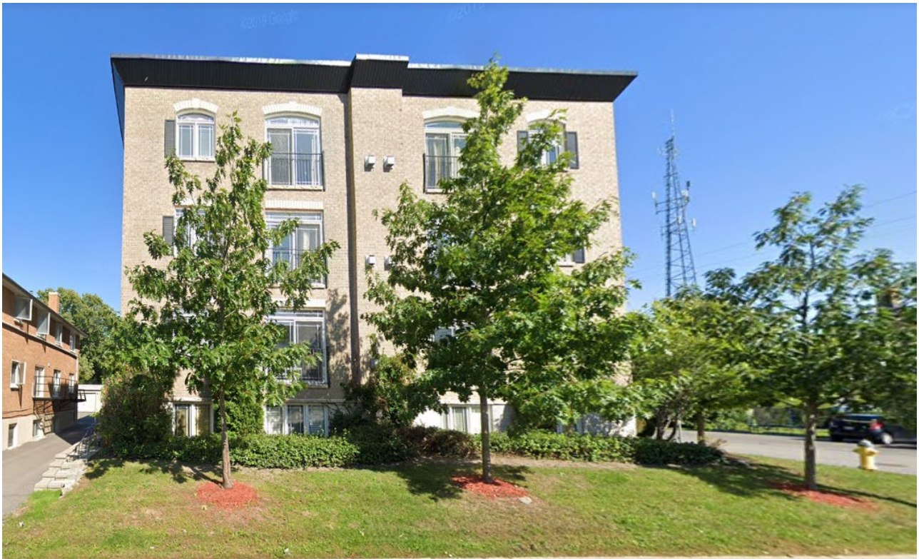
Fig. 3: A 3-storey apartment building on Churchill Avenue near Carling Avenue. It is larger in size and form than what is encountered on local streets in Westboro, however retains space for landscaping and street trees.
