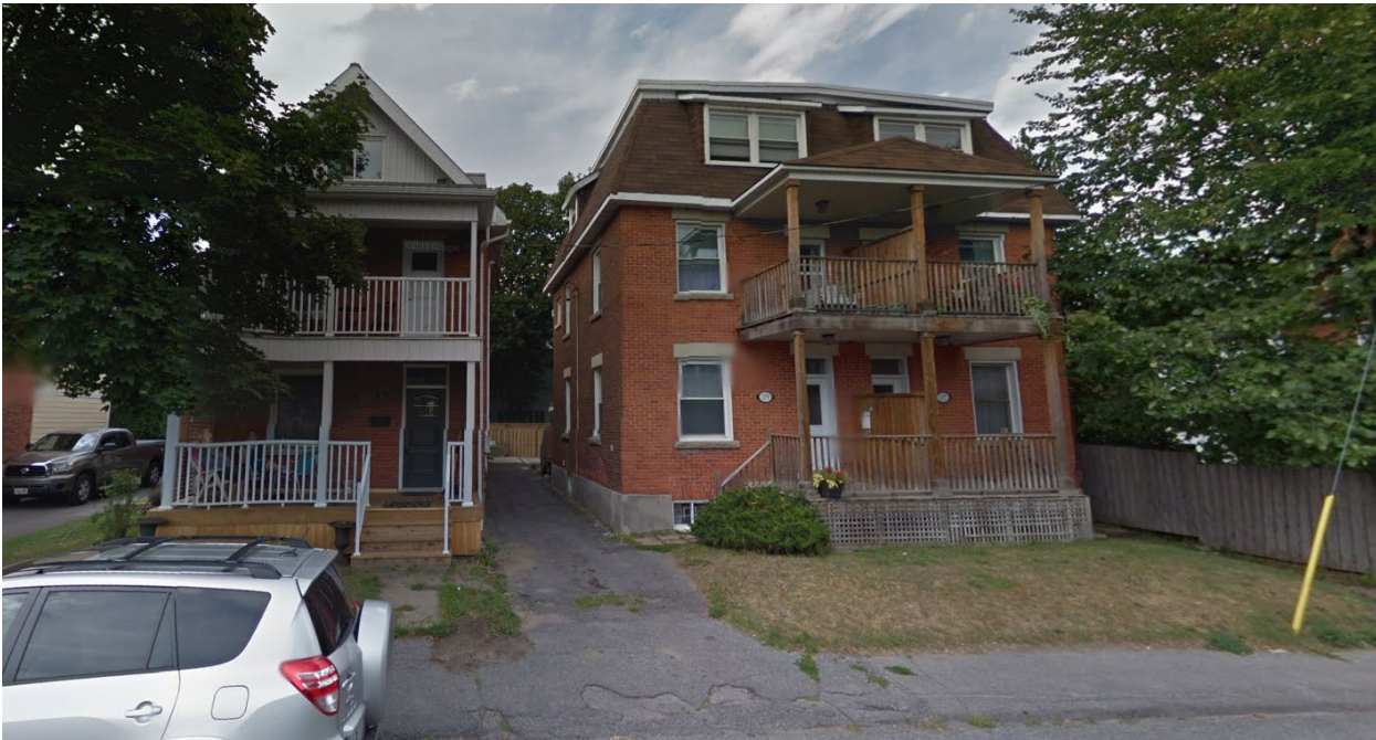
Fig. 6: The building on the right is a 6-unit building located on Wesley Avenue in the Interim Control Area, adjacent to a detached dwelling. It is three storeys in height, but is also located in close proximity to Byron Avenue, a major street within the study area, and avoids a flat roof design to mitigate the potential massing impacts of the third storey. As with the previous example, it would not be permitted under the present R3R zoning.
