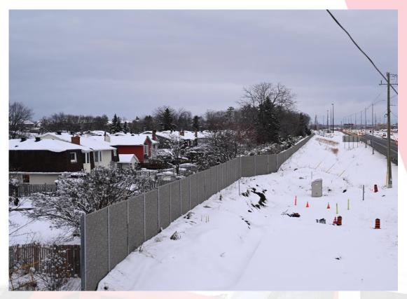
Shown is a photo of Noise Wall B03, which demonstrates an example of a completed noise wall on the north side of the OR 174. We are installing over 4.5 kms of noise walls in the East as part of the Stage 2 LRT Project.
