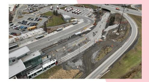
Crews completed the full civil engineering scope of the guideway construction, earthworks, drainage, overhead catenary system (OCS) foundations, sub-ballast, and ballast, and handed it over to the contractor responsible for installing track.
