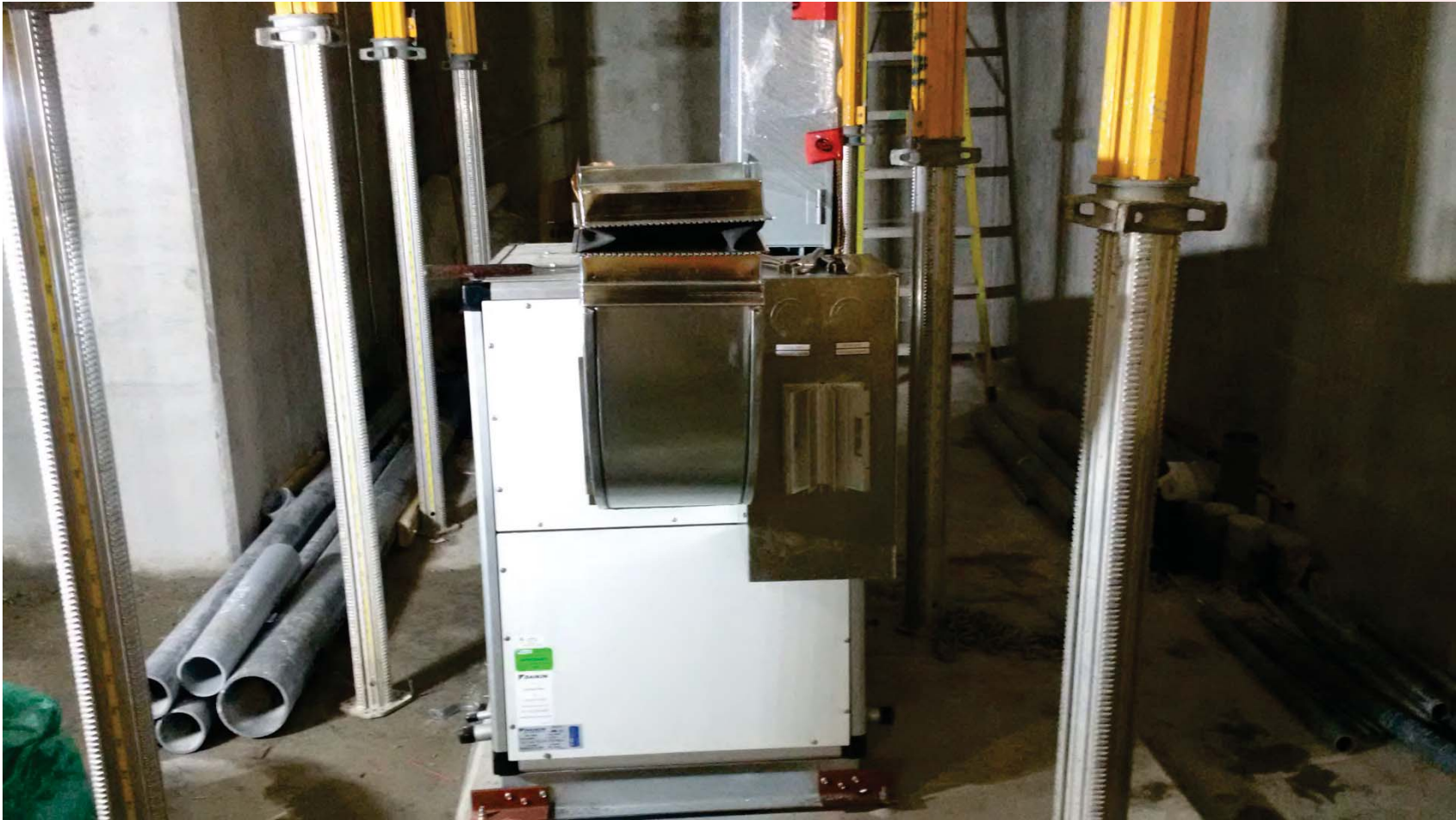
Make up air unit(Air circulation device)
