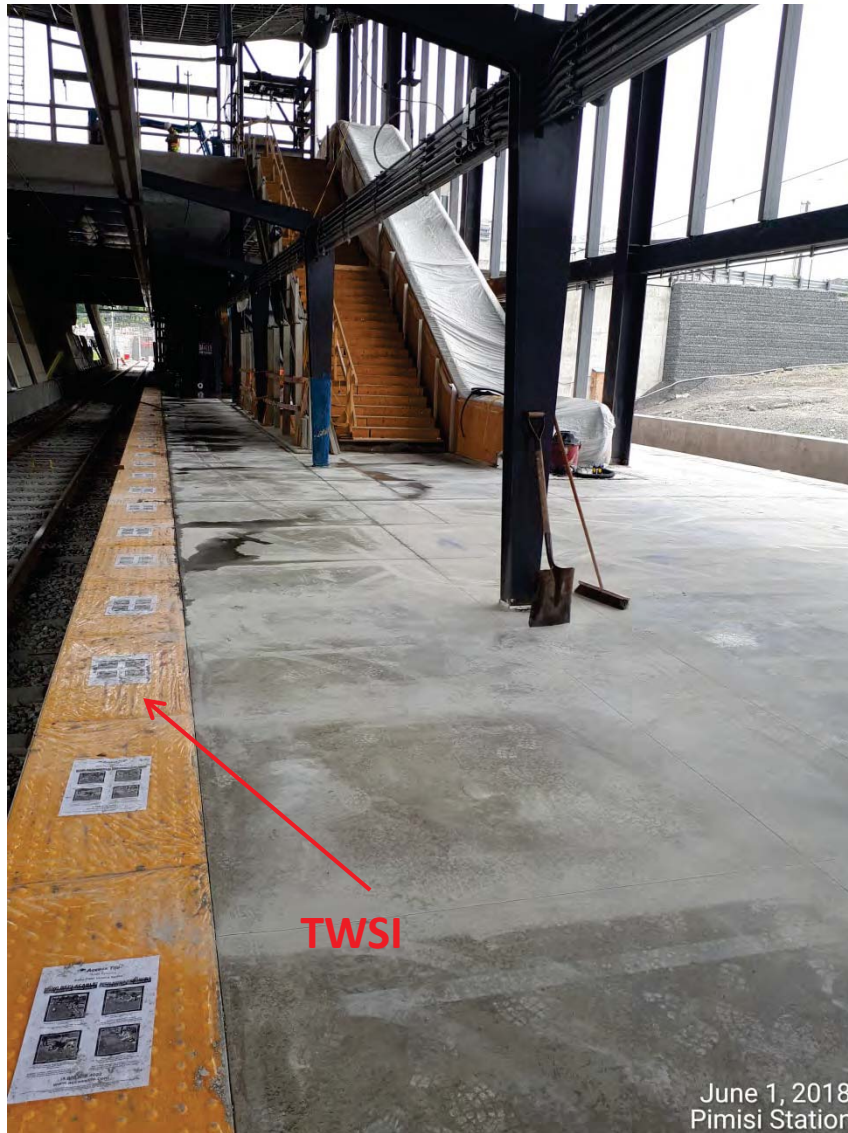
Platform West End - Conc. Topping & Saw-Cuts (50% Complete)
