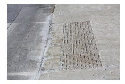
Install Accessibility for Ontarian with Disability Act (AODA) approved high tonal tactile surface. Although the colour of the tactile surface is not specified in AODA, the common high contract colour standard for most jurisdictions in North America is yellow.
