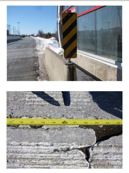
Remove the concrete barriers with a blunt end. Install drivable delineators along the base of the building on a 200 mm white line to keep buses away the station and allow the bus to remain in the departure lane. Alternatively, remove the concrete barriers and install a low concrete curb against the base of the station. In either case remove the concrete barrier with the blunt end as it is a hazard.
