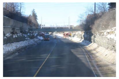
Low sun angles cannot be easily mitigated. Driver training, reduced speed and a higher level of winter maintenance are suggested for the short term. In the longer-term better drainage and a flashing beacon activated by a road surface sensor monitoring conditions such as ice and temperature are suggested.
