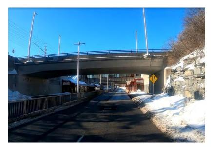
In the eastbound direction, there is no merge warning sign to warn drivers of the need to merge as the right lane ends and tapers into the left lane.
