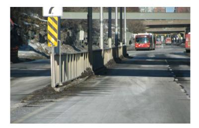
Replace the median fencing with a TL-3 F-Shape 810mm concrete barrier and TL-3 crash cushion end treatments.
