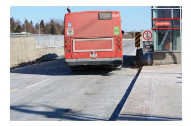
Remove the concrete barriers with a blunt end. Install drivable delineators along the base of the building On a 200 mm white line to keep buses away the station and allow the bus to remain in the departure lane. Alternatively install a low concrete curb against the base of the station.
