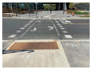
Markings from a previous configuration were black-masked, contrary to City of Ottawa standard practices. The black paint has since worn off, causing the older crosswalk markings to show through. The most recent markings have also worn/faded, making them similar in appearance to the old markings. This has rendered the resulting visible markings non-standard, which could contribute to user confusion.
