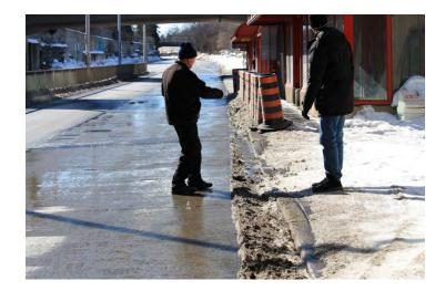
Replace the letdown curb on the approach end of the station platform with a 150mm high barrier curb. The letdown curb on the departure end of the station platform can remain.
