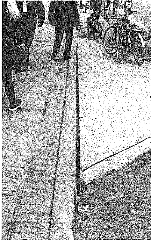
Figure 9-3:47-57 Rideau Street Sidewalk/Curb Separation Photo (June 6, 2016)
