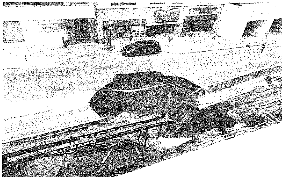
Figure 1-2: Sinkhole on Rideau St. Looking North at 47-57 Rideau St
