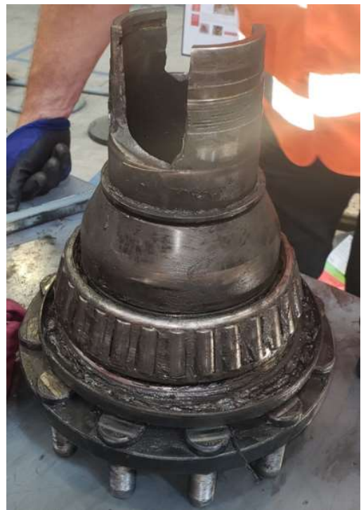
Figure 3. Light rail vehicle 1127 failed axle hub (Source: TSB)
