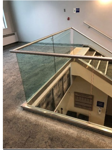
Example 4-Free-standing glass guard (continuous shoe) with top rail.
