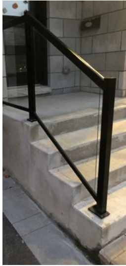
Example 1-Glass in guard with continuous top and bottom support.
