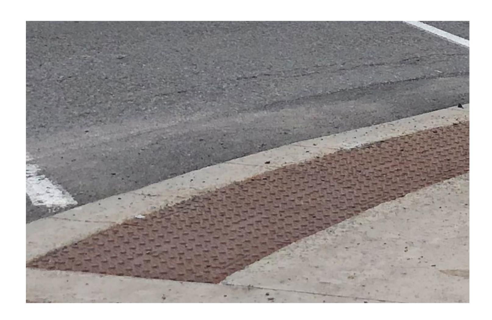
TWSI are plates installed level with the concrete that are meant to be detectable underfoot or with a cane. They are used to warn people of a potential hazard such as a roadway.
