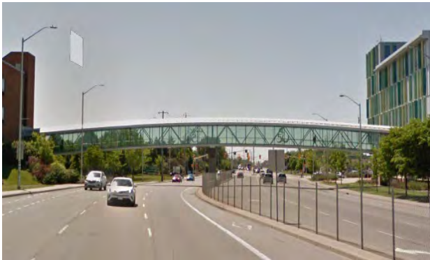
Figure 3-13 Pedestrian bridge across Woodroffe Avenue looking south
