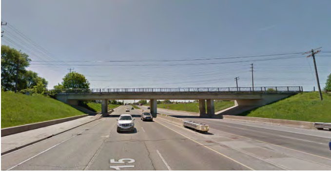
Figure 3-18 CN Rail line overpass of Woodroffe Avenue
