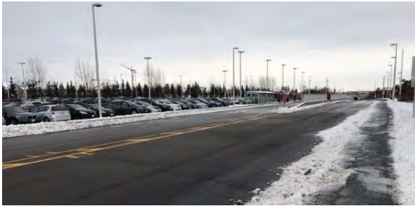
Figure 3-31 MUP located to the east of the Southwest Transitway underpass at Highbury Park looking south
