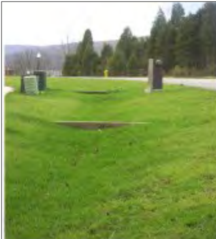
Figure 7-11 Enhanced Grass Swale with Check Dams (TRCA, 2016)
