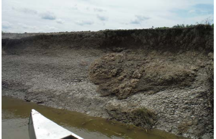
Stream bank erosion with visible soils and lack of vegetation
