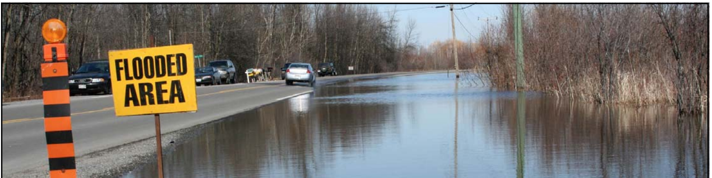
Flooded road section in the Stevens Creek catchment near the Rideau River
