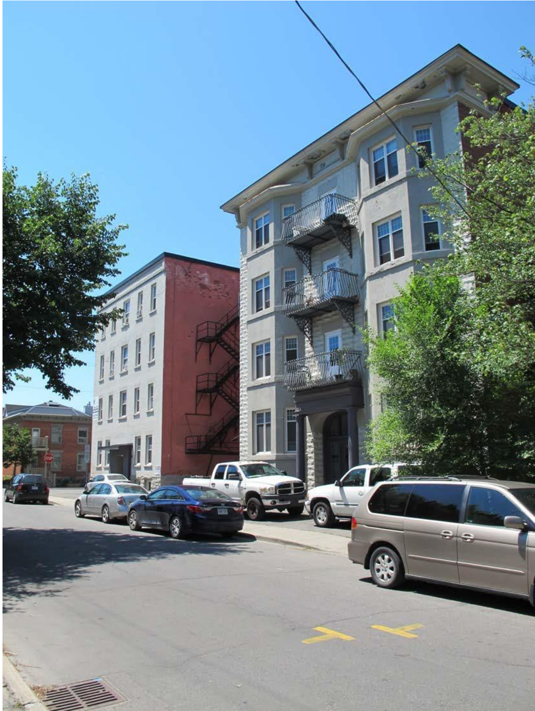
Fig. 11: Fire escapes on side of building (Daly)
