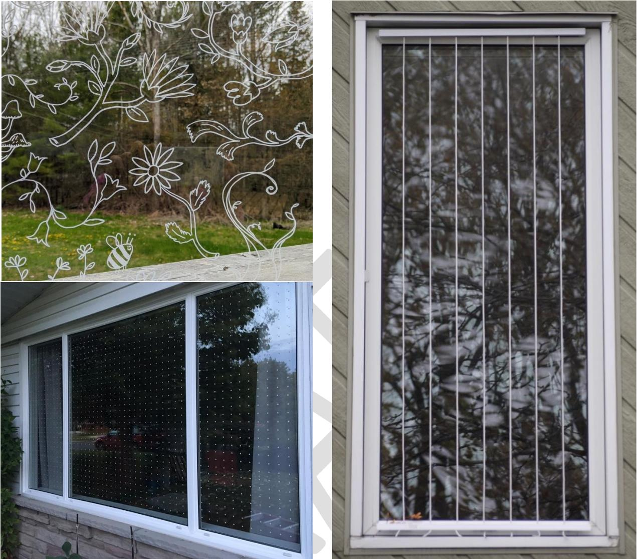
Figure 11: Examples of window treatments (oil-based paint marker mural top left, Feather Friendly DIY tape bottom left, Acopian BirdSaver on right). Photos courtesy of Kate Stolwyk, Karen Gordon and Safe Wings Ottawa, respectively.
