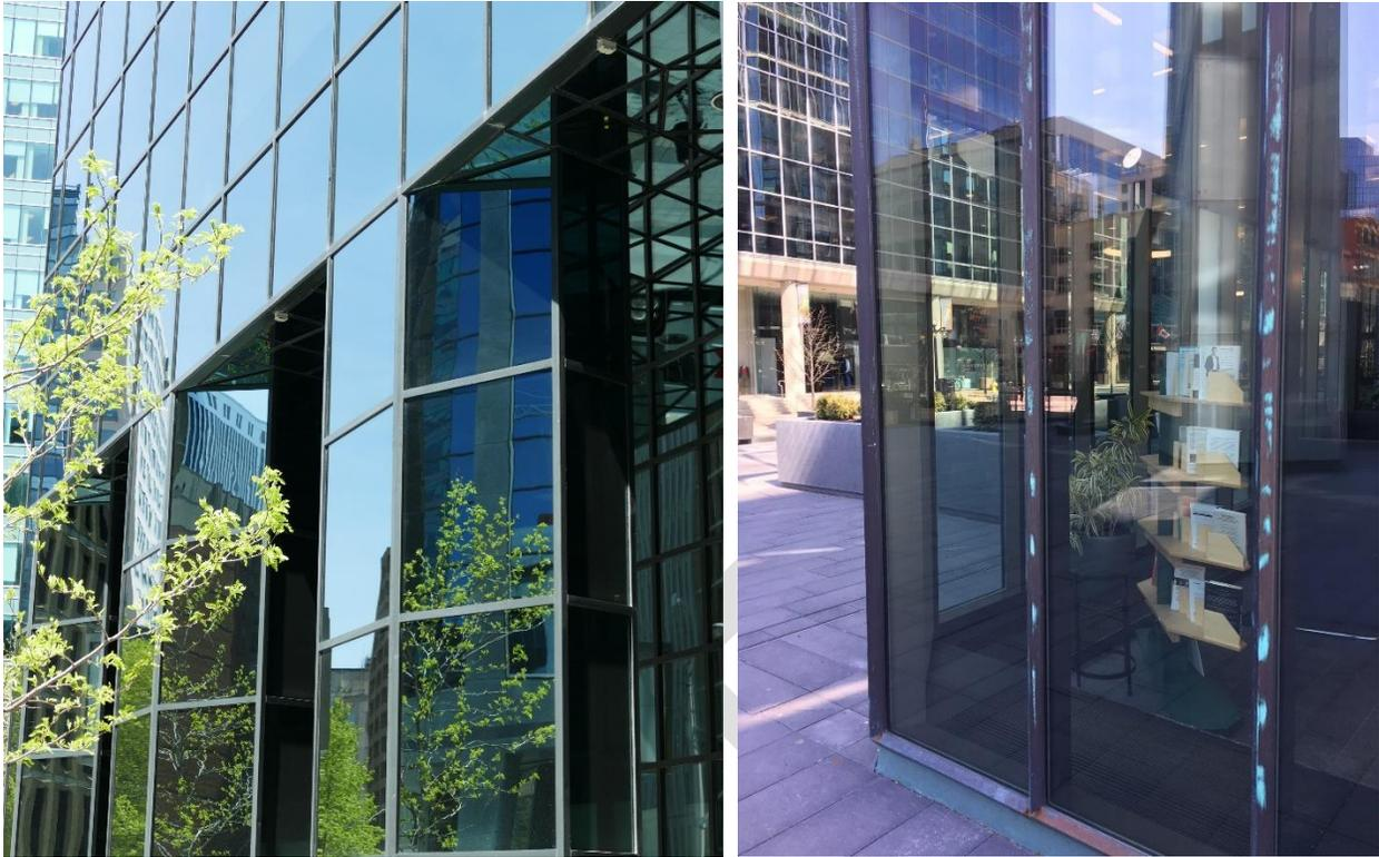
Figure 8: Potential design traps (mirror maze and black hole effect on left, corner glass on right).
