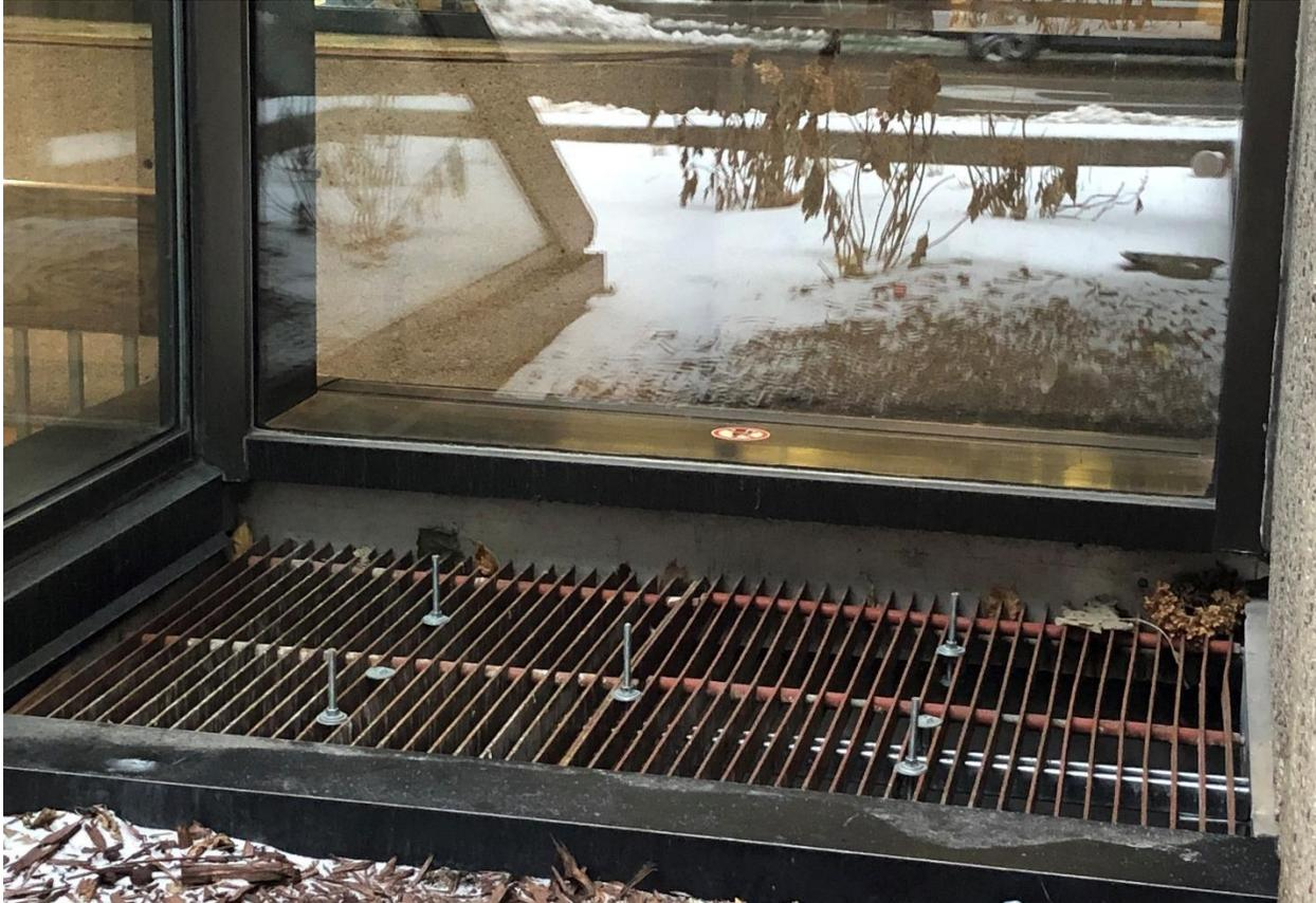
Figure 9: Open grate beneath reflective glass windows.
