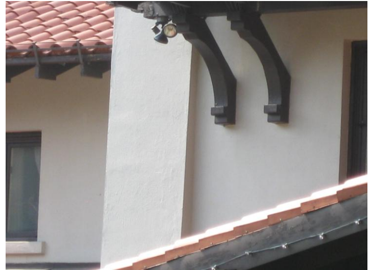
FIGURE 29: SMOOTH STUCCO CLADDING AT 85 GLEBE AVENUE
