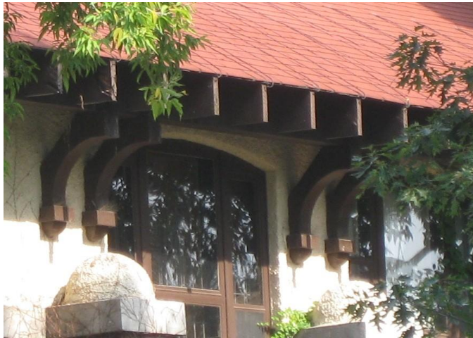
FIGURE 35: WOOD EAVES BRACKETS
