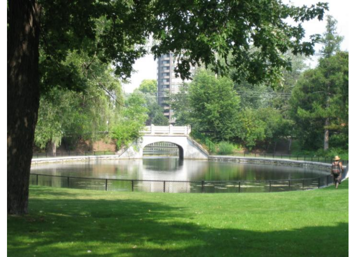
FIGURE 25: PATTERSON CREEK AND O'CONNOR STREET BRIDGE
