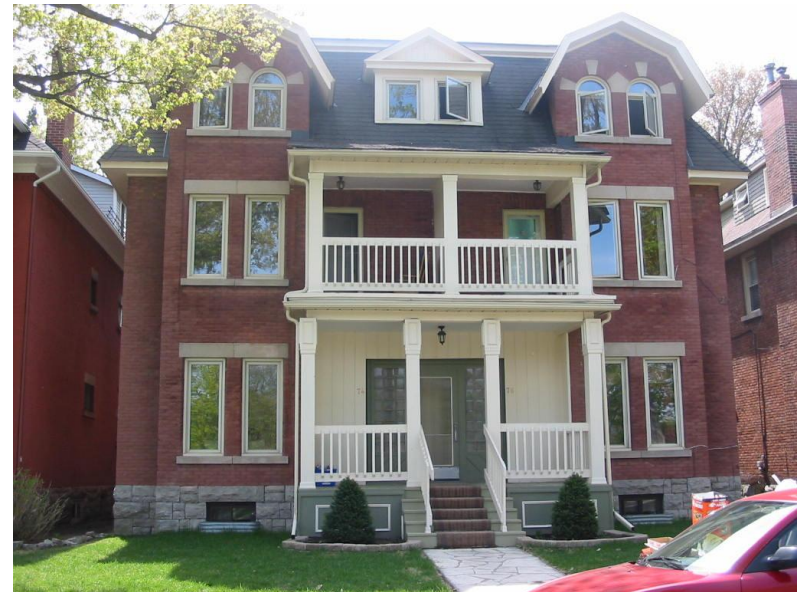
FIGURE 37: CATEGORY 3 BUILDING AT 74-76 GLEBE AVENUE
