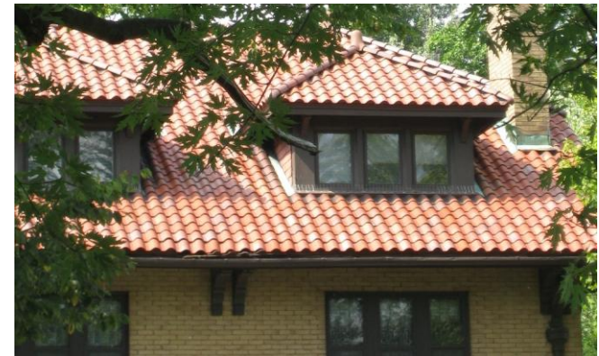
FIGURE 28: CLAY TILE ROOF
