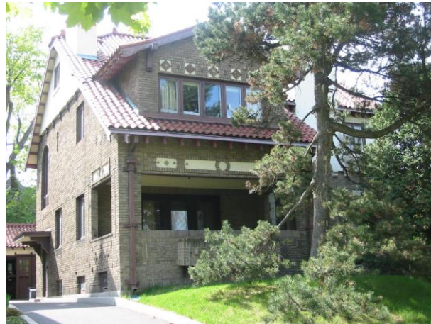
FIGURE 33: PORCH ON CLEMOW AVENUE
