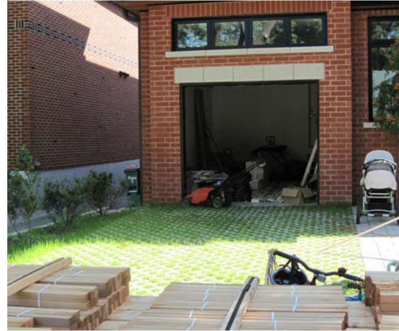
Figure 29: Turf block provides a stable base for parking while increasing on-site infiltration of surfacewater.
