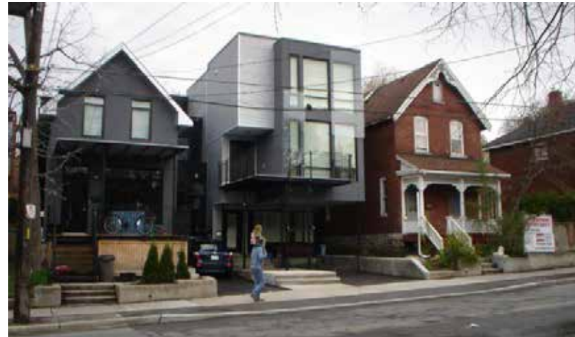
Figure 21: This semi-detached infill unites two different architectural styles. The renovated unit on the left is attached to the contemporary middle unit but reflects the form and character of the existing single-detached red brick home. The contemporary unit adopts the colours of the renovated unit to blend into the streetscape.
