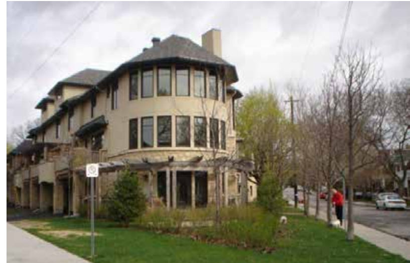
Figure 17: The curved façade, echoed by the curved arbour, creates a unique corner treatment that adds interest to the public realm. The significant glazing contributes to community surveillance.
