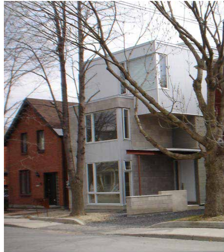
Figure 9: This urban infill matches the setbacks of surrounding homes and preserves an established tree. The front door faces the street, the ground floor elevation matches that of the neighbours and the large first floor window contributes to an animated and safe street.
