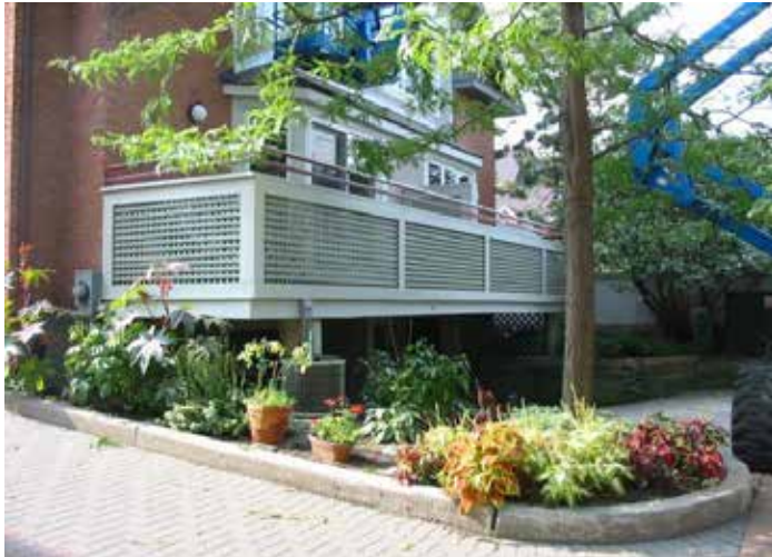
Figures 12 and 13: These two rows of infill townhomes, built around an internal parking court, use extensive landscaping to enhance the development. Generous balconies predominate over recessed garages.
