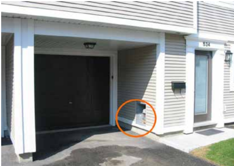
Figure 31: Service elements are integrated into the design of this home by making them visually less prominent.
