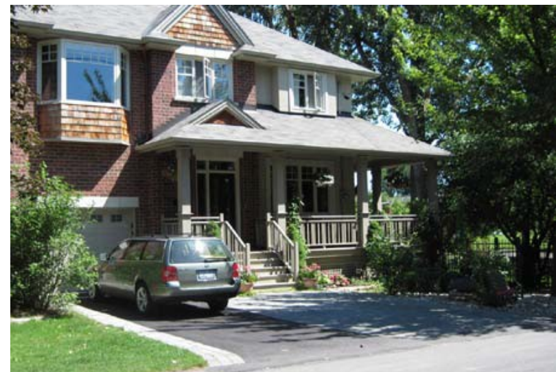
Figure 19: A covered porch articulates the front façade and highlights the entrance to this home.
