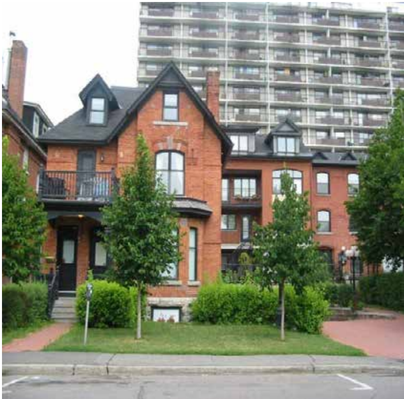
Figure 30: The red brick infill addition, which is set back and to the right of this neighbourhood building, blends into the existing context through its compatible composition, materials and colours. Its placement on the site showcases the heritage building.
