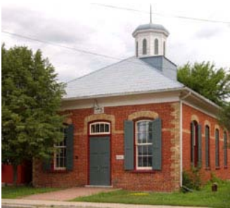
Figure 18: Architectural features such as a door transom, lintels, window muntins, quoins and materials show the character and history of this former town hall, from in 1876 (North Gower).
