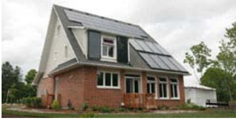
Figure 25: Photovoltaic solar panels, on-site rainwater collection and natural ventilation are just some of the sustainable features incorporated in Minto's eco-home (Manotick). *Examples of green building and energy rating standards include LEED Canada for Homes, Energy Star or R2000 construction.
