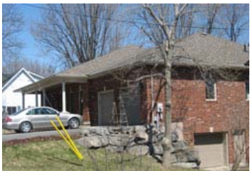
Figure 3: The design of a home takes advantage of an existing, natural change in grade (Kars).
