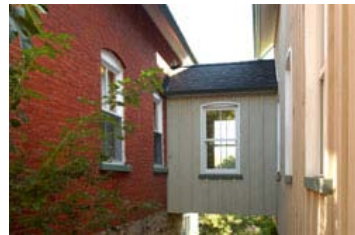
Figure 24: An innovative residential connection bridges an old building with a new building using complimentary colours and durable materials (Manotick).
