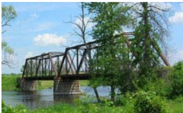
Figure 14: Preserving important views and iconic cultural landscapes, such as a historic bridge, contributes to a unique community identity (Galletta).
