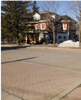
Figure 35: Crosswalks and sidewalks in a village core contrast the roadway and help define the pedestrian area (Vars).
