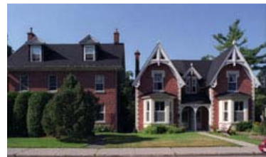
Figure 5: Two semi-detached houses avoid a "cookie cutter" look by having varied designs. The designs also integrate well with the detached homes along the block (Ottawa).
