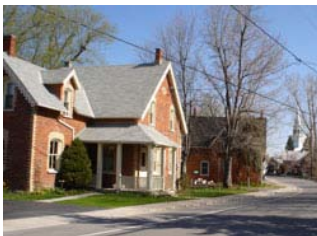
Figure 28: A wrap-around porch on a heritage building visually divides the front façade (North Gower).
