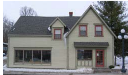
Figure 23: A commercial addition uses the same materials, colours and trims to complement original building (Carp).
