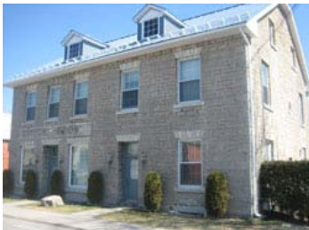
Figure 9: A heritage building provides multi-unit housing in the village core. Having a range of residential densities close to amenities and services provides choice and convenience for village residents (Richmond).
