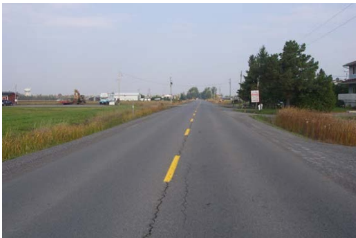
Mer Bleue Road looking north
