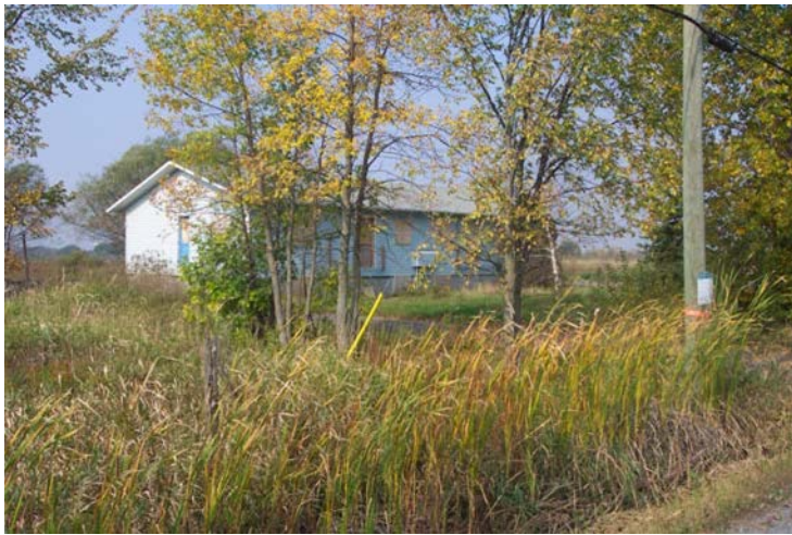
Unoccupied dwelling along Tenth Line Road
