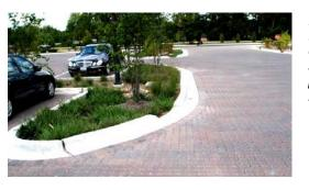
Figure 51b: Planting islands with depressed curbs allow stormwater to run from paved areas into the islands.
