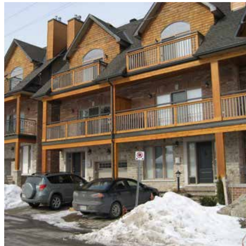
INFILL HOUSING AT STONEHURST AND LYNDALE AVENUES
