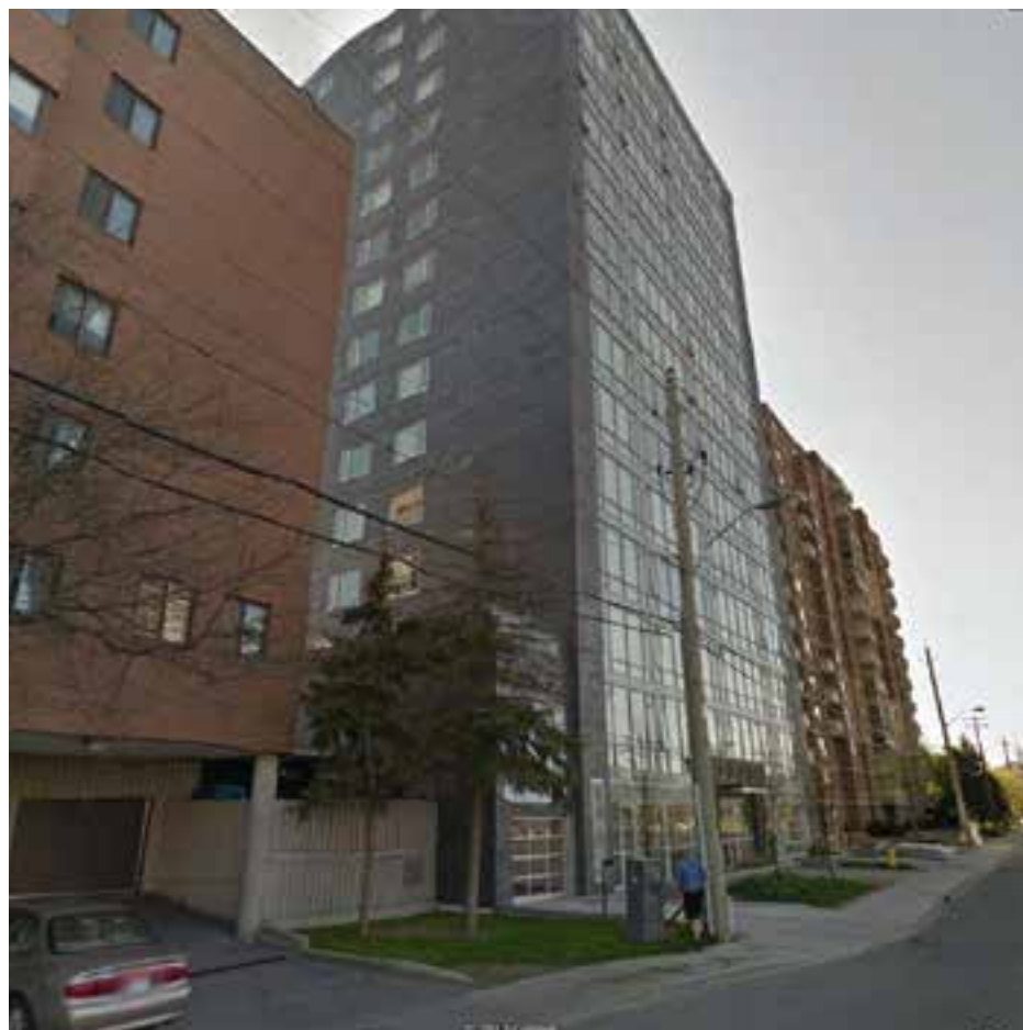
SOHO DEVELOPMENT ON PARKDALE AVENUE
