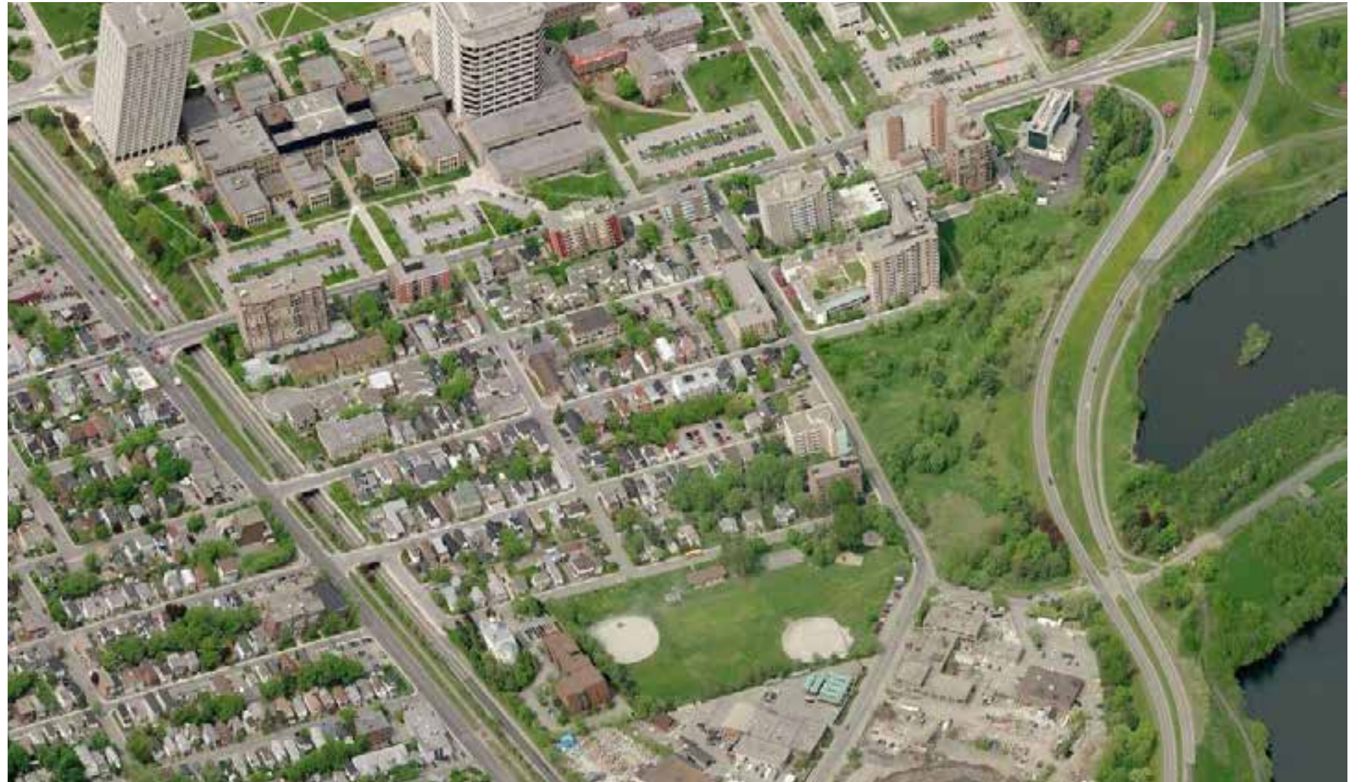
AERIAL OF MECHANICSVILLE
