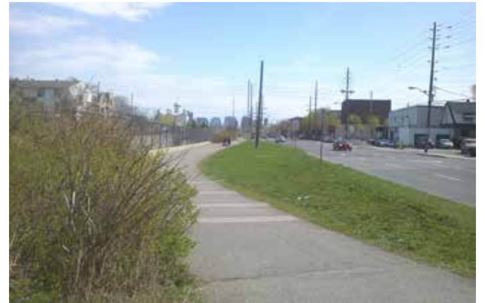
EXISTING MULTI-USE PATH - SCOTT STREET
