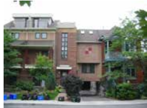
Figure 52: There is one common access point to the parking area in this multi-unit building.
