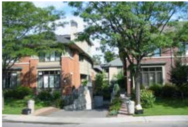
Figure 20: Communal access to a parking area. There are no garages facing the street.
