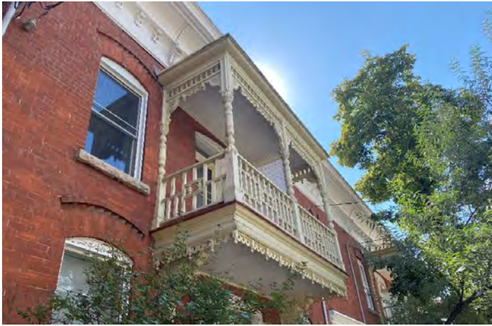
Figure 41: Cantilevered balcony at 208 St. Patrick Street.
