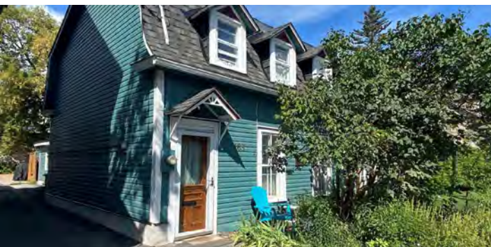
Figure 29: Wood siding at 163 Bolton Street.
