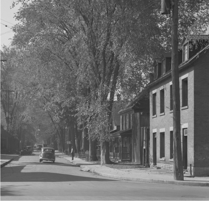
Figure 50: Guigues Avenue at King Edward, n.d. Credit: Library and Archives/ 4101933.
