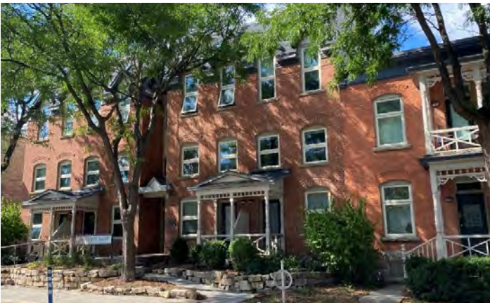
Figure 46: Example of compatible new construction on St. Patrick Street.
