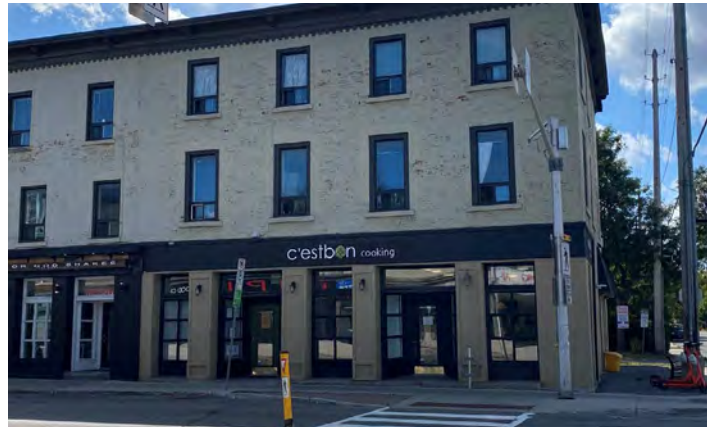
Figure 36: Storefronts on Dalhousie.
