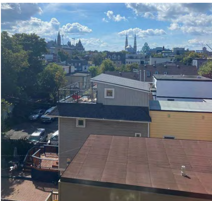
Figure 45: Example of roof top addition at the rear of a property.
