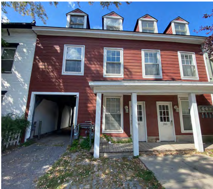
Figure 42: Carriageway on Bruyère Street.
