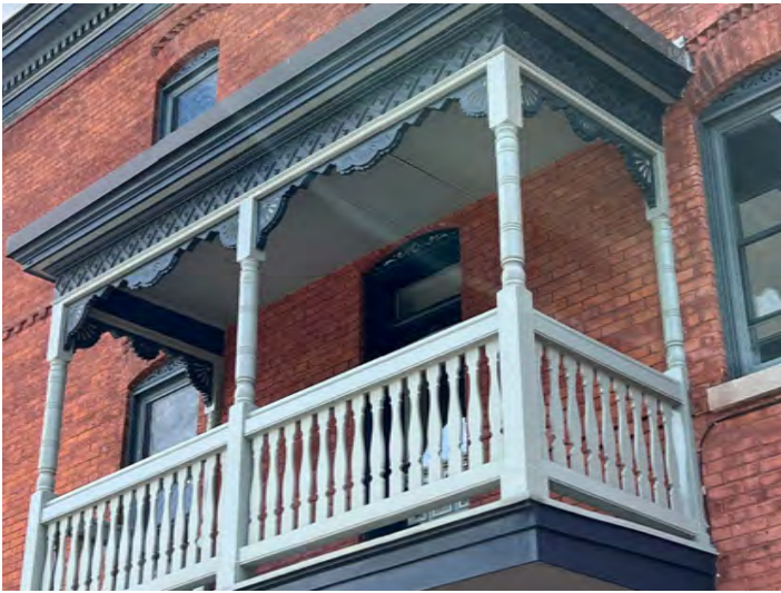
Figure 35: Balcony with decorative trim.
