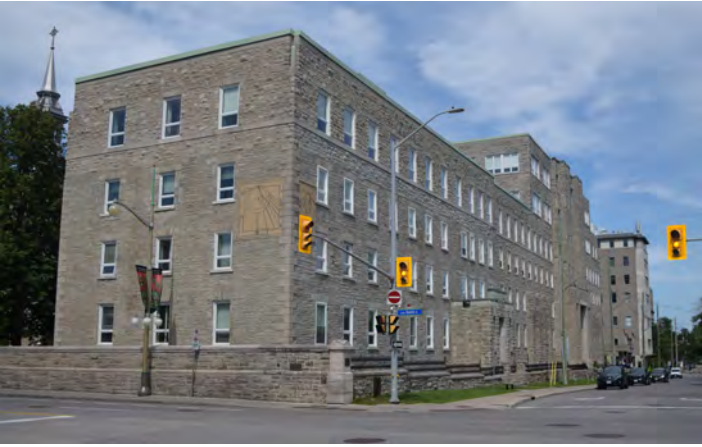
Figure 20: Elisabeth Bruyère Hospital at 9 Bruyère Street, formerly the Grey Nuns Mother House.
