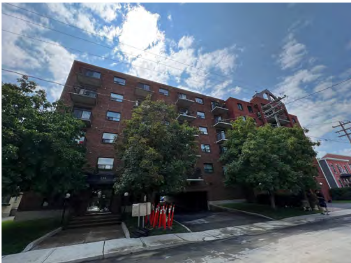
Figure 24: Non-contributing property in the HCD.
