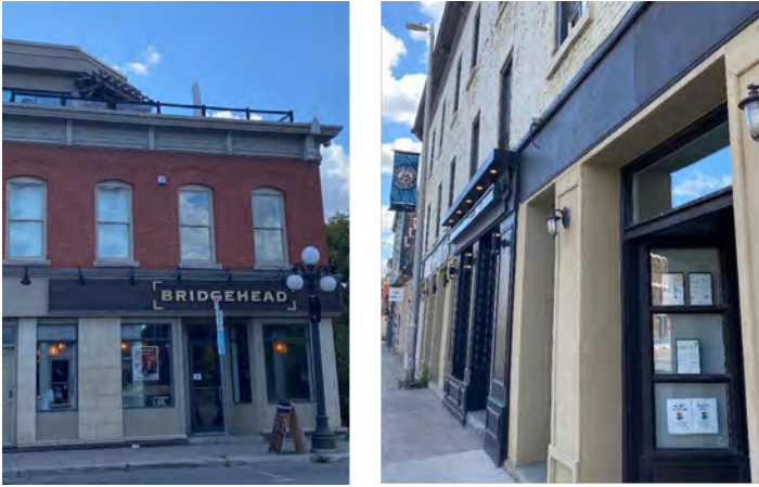
Figure 53: Examples of sensitive corporate signage and lighting (left) and downlighting (right).
