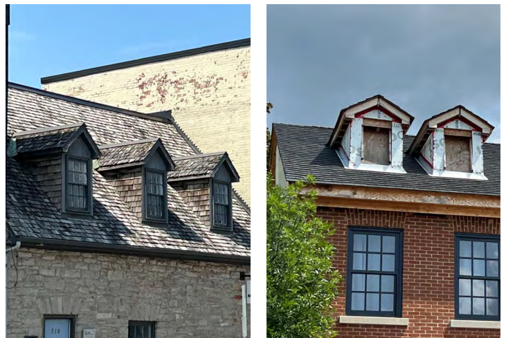
Figure 38: Existing and new dormers in the HCD.
