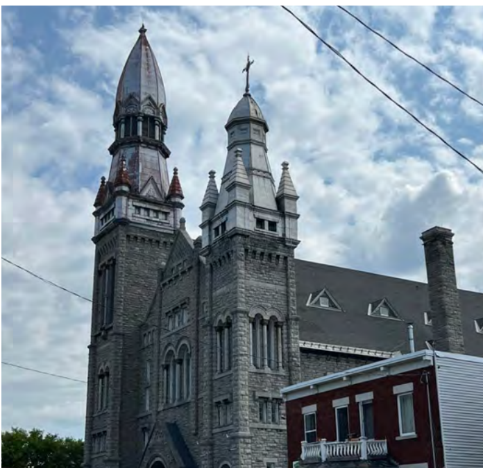
Figure 21: Former St. Brigid’s Church.
