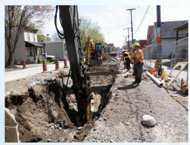
Sewer installation with one lane traffic and pedestrian access
