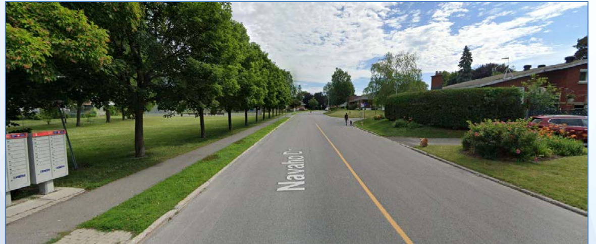
Navaho Drive facing eastward at Laxton Crescent
