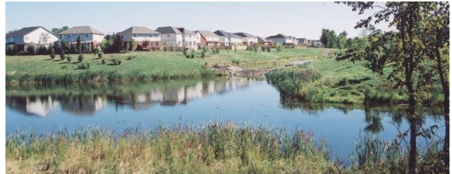
Figure 5: Storm Water Management Pond
