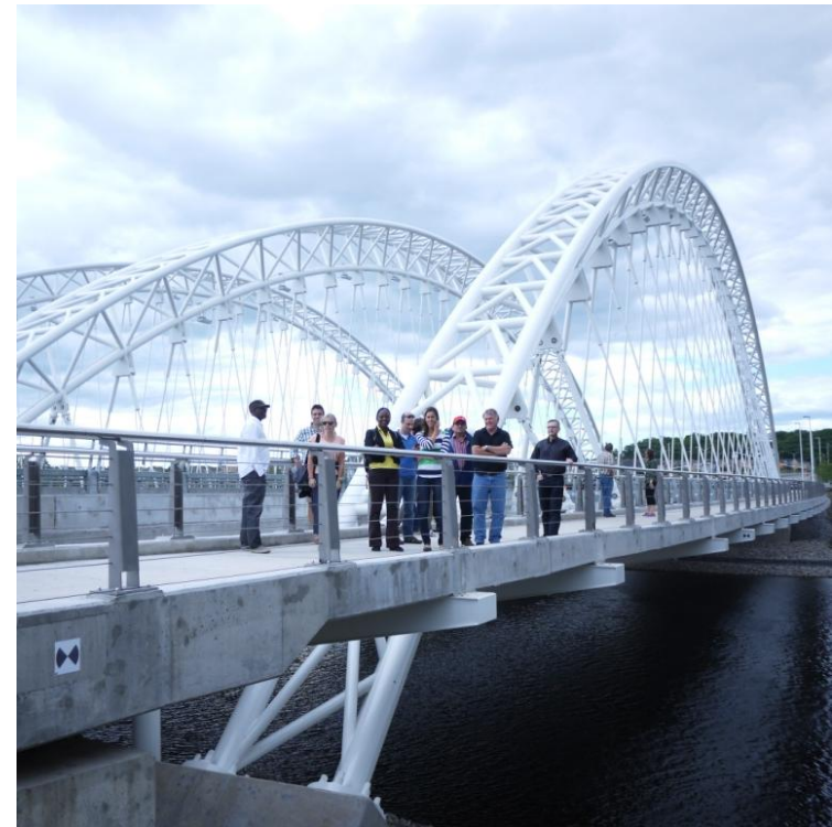
Figure 44: The Vimy Memorial Bridge
