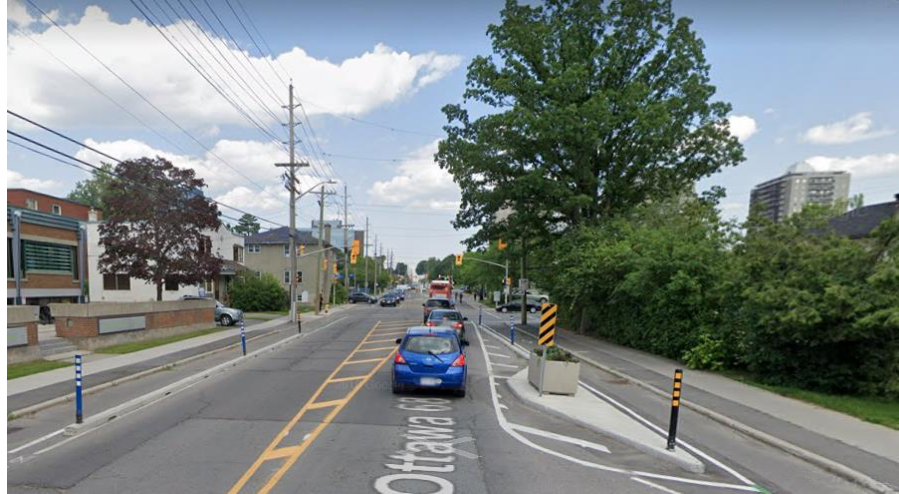
Example of pinned curb separated cycling facility on McArthur Ave
