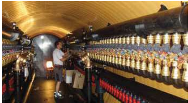
Distribution components in the distribution shaft
